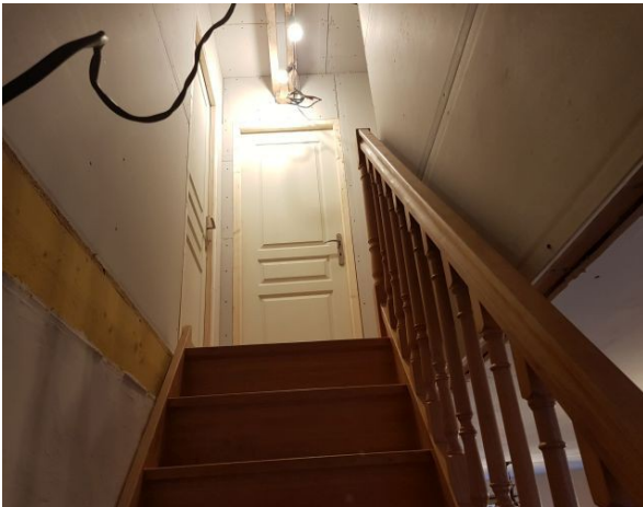
Onto the landing/ bedroom door ahead Door to recreation area on left
