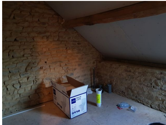
Bathroom waiting for the sanitary ware to be installed
