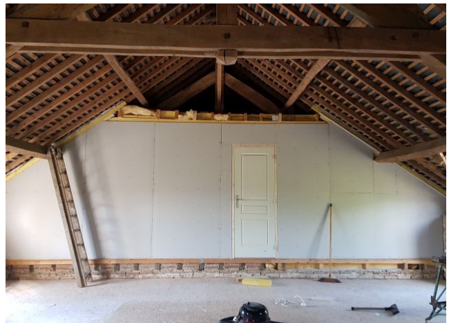
Finished back wall in recreation area
