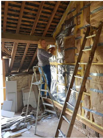
Insulating the back wall
