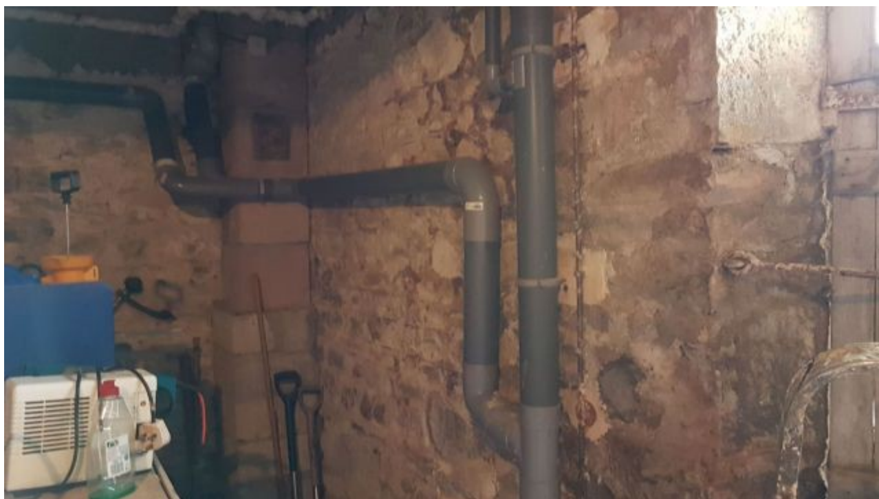
Finished plumbing in workshop before I replaced the lagging
