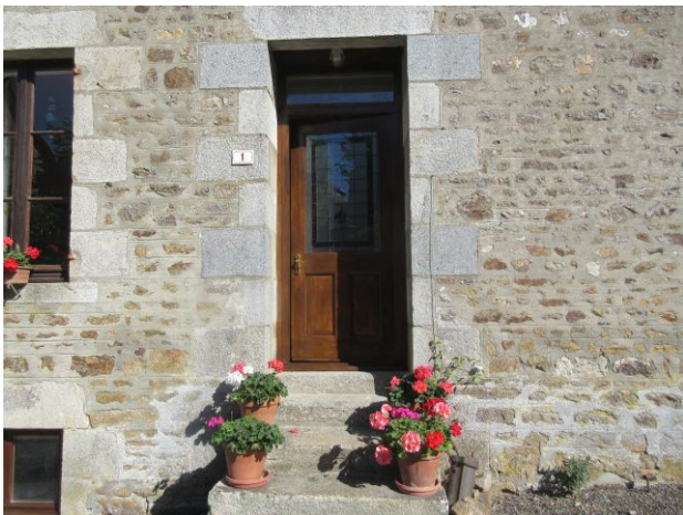
The finished door
