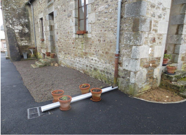
Temporary rainwater fix
