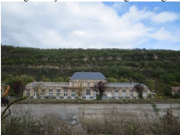
The disused Railway Station at Lexos
