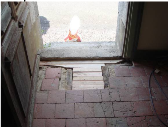
All boarded up and ready to be levelled
